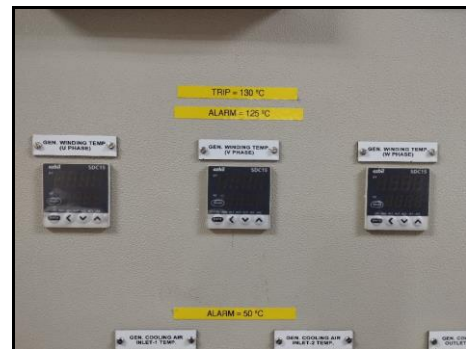
Temperature indicator for stator coils
