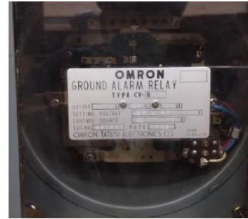
Ground over voltage relay
